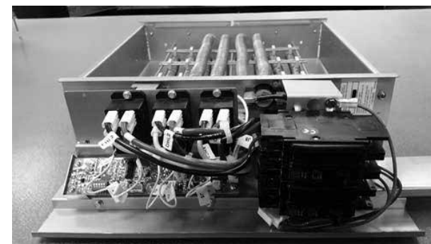
Heaters installed with reverse polarity on one of the breakers can cause the heater to overheat, posing a fire hazard.
